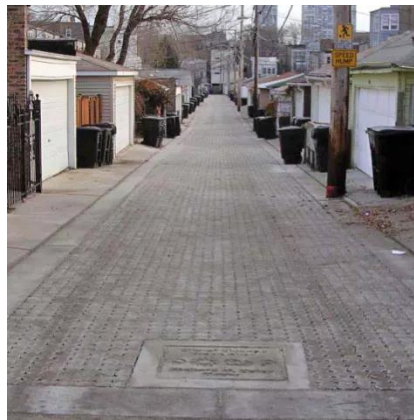
Image 2: Impermeable landscape example. A back alley with zero permeable surface - all rain water must be diverted and no soil is exposed.
